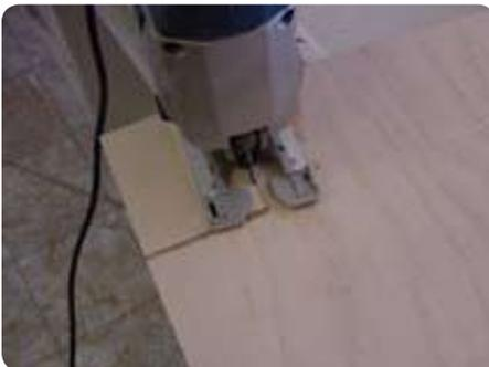
2. **Installing End Panels.** When installing end panels on lower cabinets, you may have to cut out a notch for the cabinet toe kick. Mark the back of the panel then using your jigsaw cut it out. A jigsaw cuts upward, it can cause the material to splinter. This is why it is important to cut on the back of the panel. Double check by holding the panel in place before you make your cuts.
