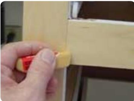
9. **Finishing touches.** Use a color putty stick to cover the nail holes on the end panel, molding and any joint that might be a little loose.
