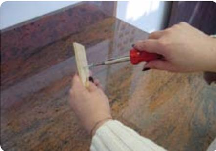
2. With a screw driver, center the screw on the piece of wood and drive all the way through.
