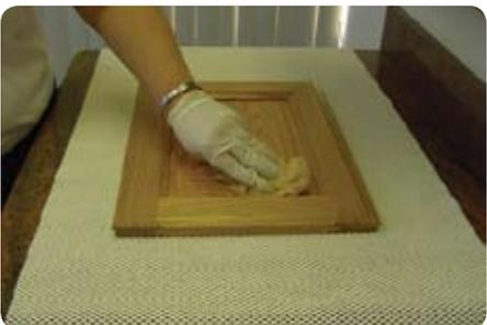
10. With a tack cloth, go over the whole door to remove fine dust and debris
