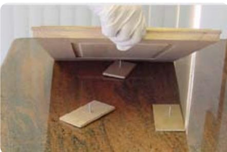
5. Lay out 3 support blocks, turn the door over, and gently lay the door on the 3 support blocks.
