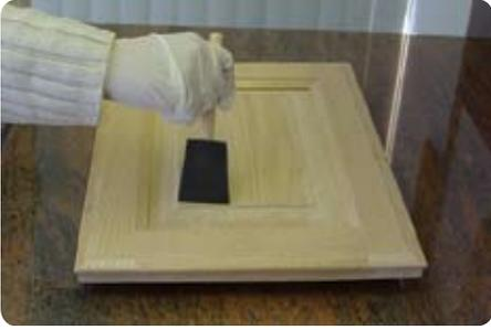
6. Apply the polyurethane as you did on the back side making sure not to press too hard. Do not over work the finish, just quickly apply a thin even coat.
